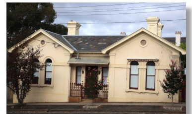
Former Gold Warden's Office
